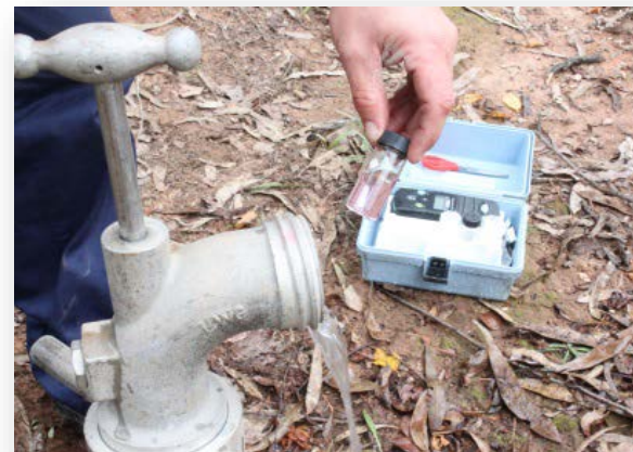
Mains flushing following a repair and a chlorine residual test being completed at nearest downstream hydrant to the repair
