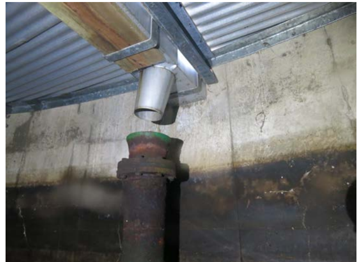
Roof drainage not effective
