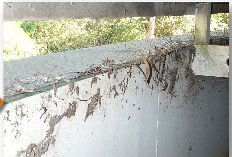
Vent mesh unsecured or unsealed
