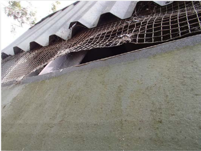
Vent mesh unsecured or unsealed
