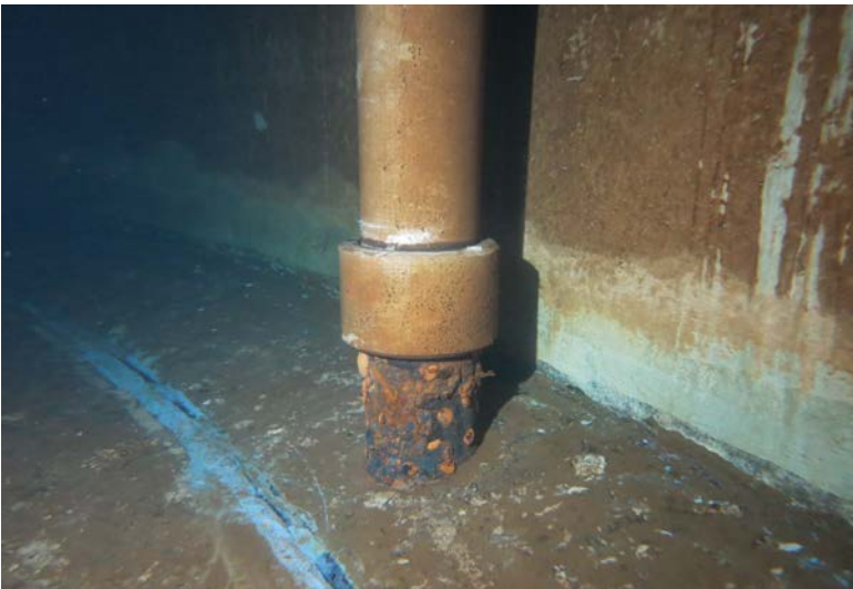
Unsuitable pipework materials – ductile iron and asbestos cement
