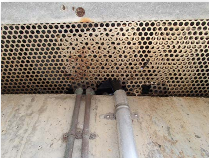
Vent mesh unsecured or unsealed
