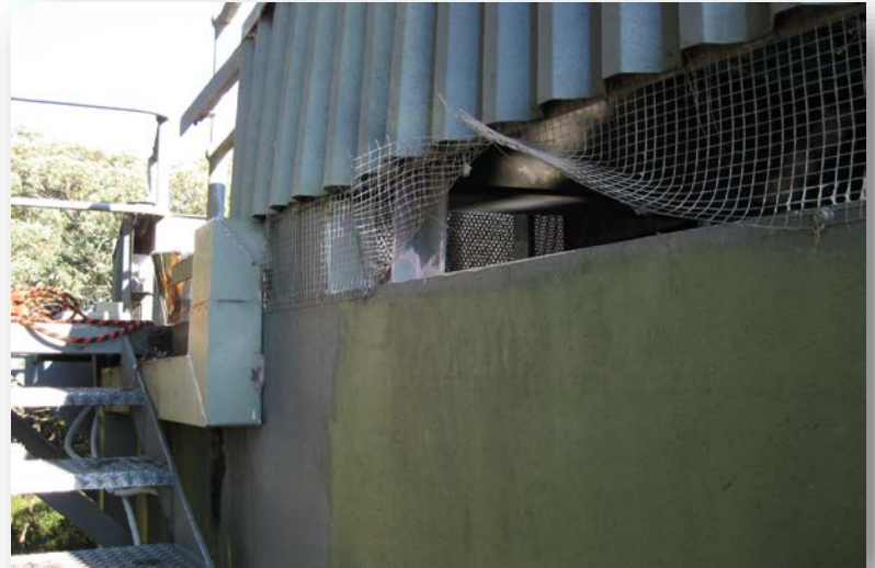
Vent mesh unsecured or unsealed
