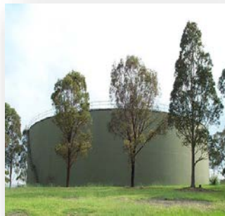
Trees starting to intrude onto storage tanks, causing roof impact damage or root intrusion
