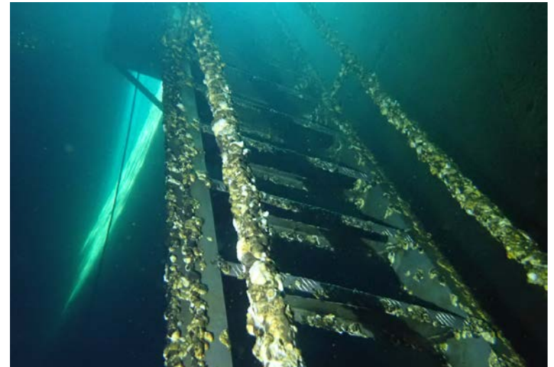
Corroded ladder structures
