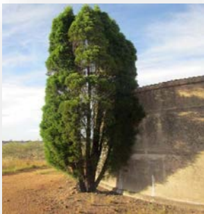
Trees starting to intrude onto storage tanks, causing roof impact damage or root intrusion
