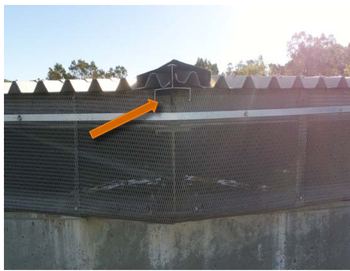
Vent mesh unsecured or unsealed
