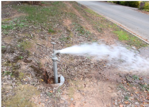
Mains flushing following a repair and a chlorine residual test being completed at nearest downstream hydrant to the repair
