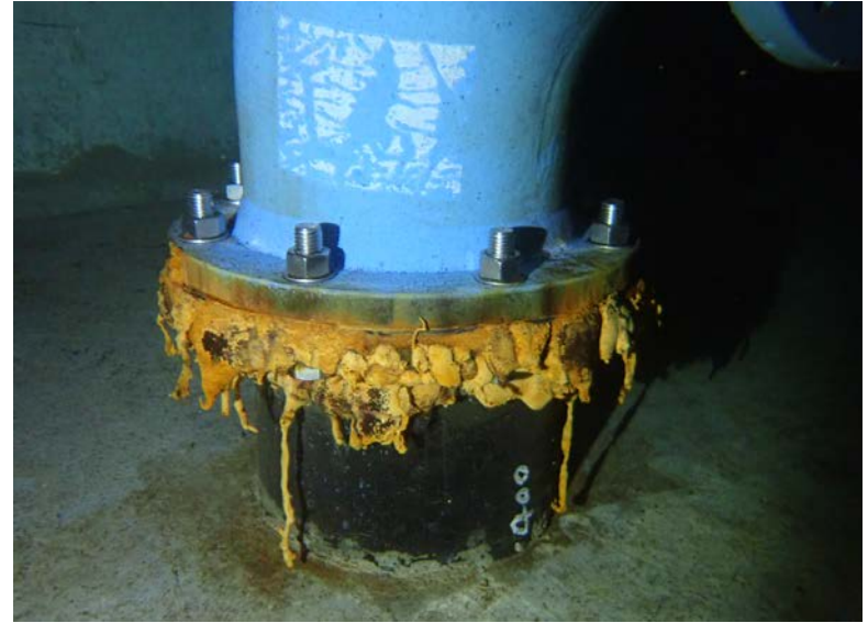
Unsuitable pipework materials – ductile iron and asbestos cement
