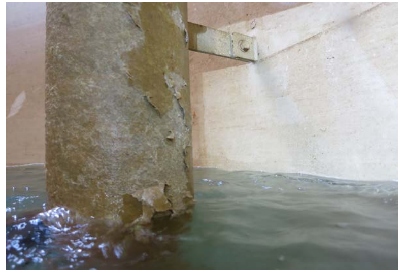
Unsuitable pipework materials – ductile iron and asbestos cement
