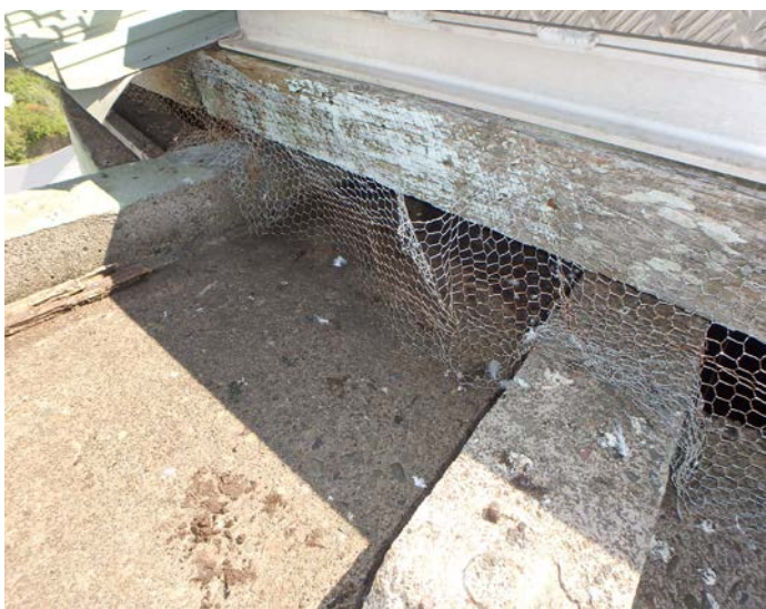
Vent mesh unsecured or unsealed
