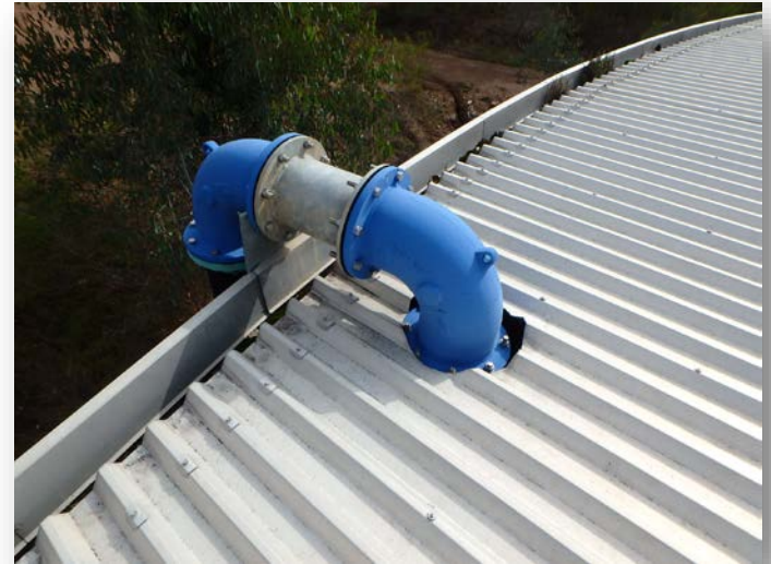
Roof pipework unsealed or not connected
