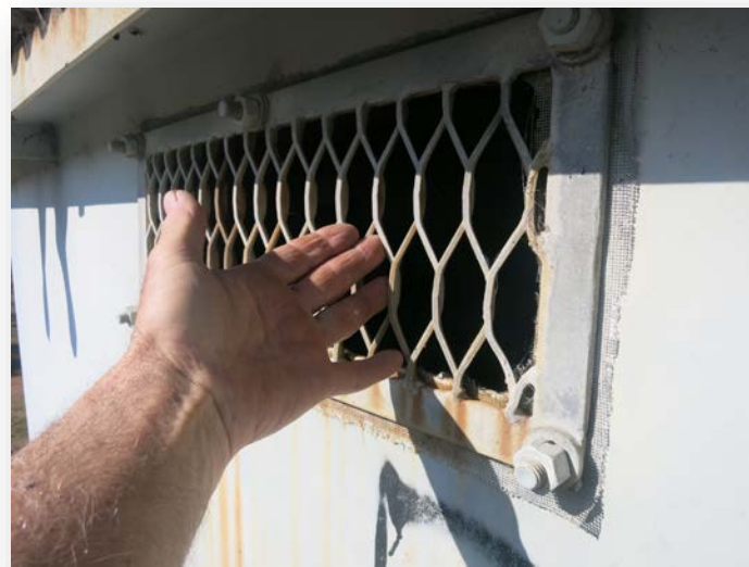
Vent mesh unsecured or unsealed
