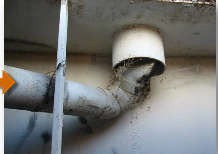
Roof pipework unsealed or not connected
