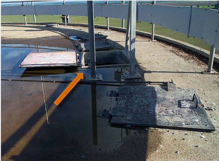
Roof drainage not effective
