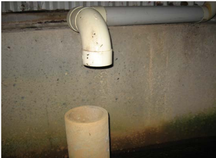
Roof drainage not effective
