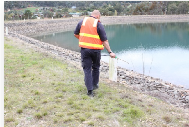
Decanting weed killer and spraying directly adjacent to a raw water or clear water storage
