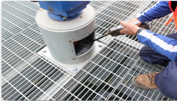
Grease gun being used directly over a treated water storage
