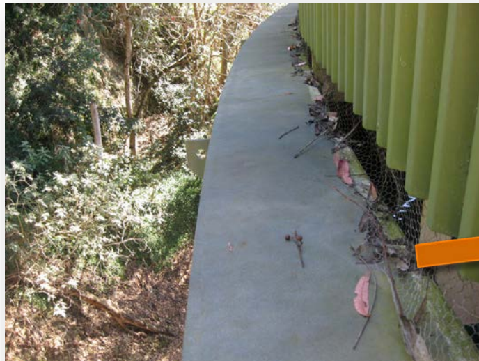
Vent mesh unsecured or unsealed
