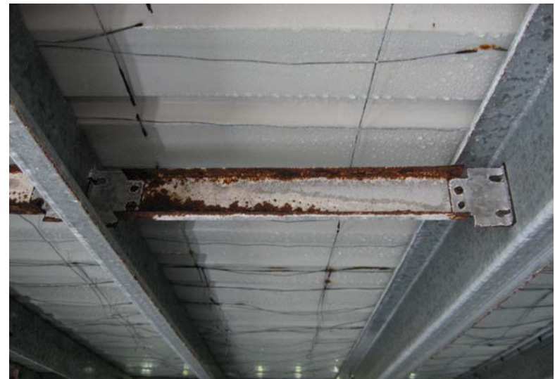
Poor roof framing materials
