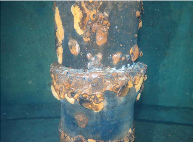
Unsuitable pipework materials – ductile iron and asbestos cement
