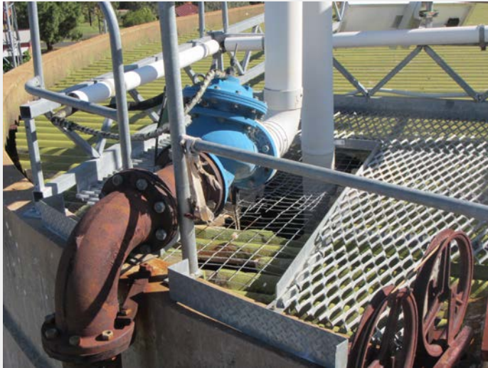
Roof pipework unsealed or not connected
