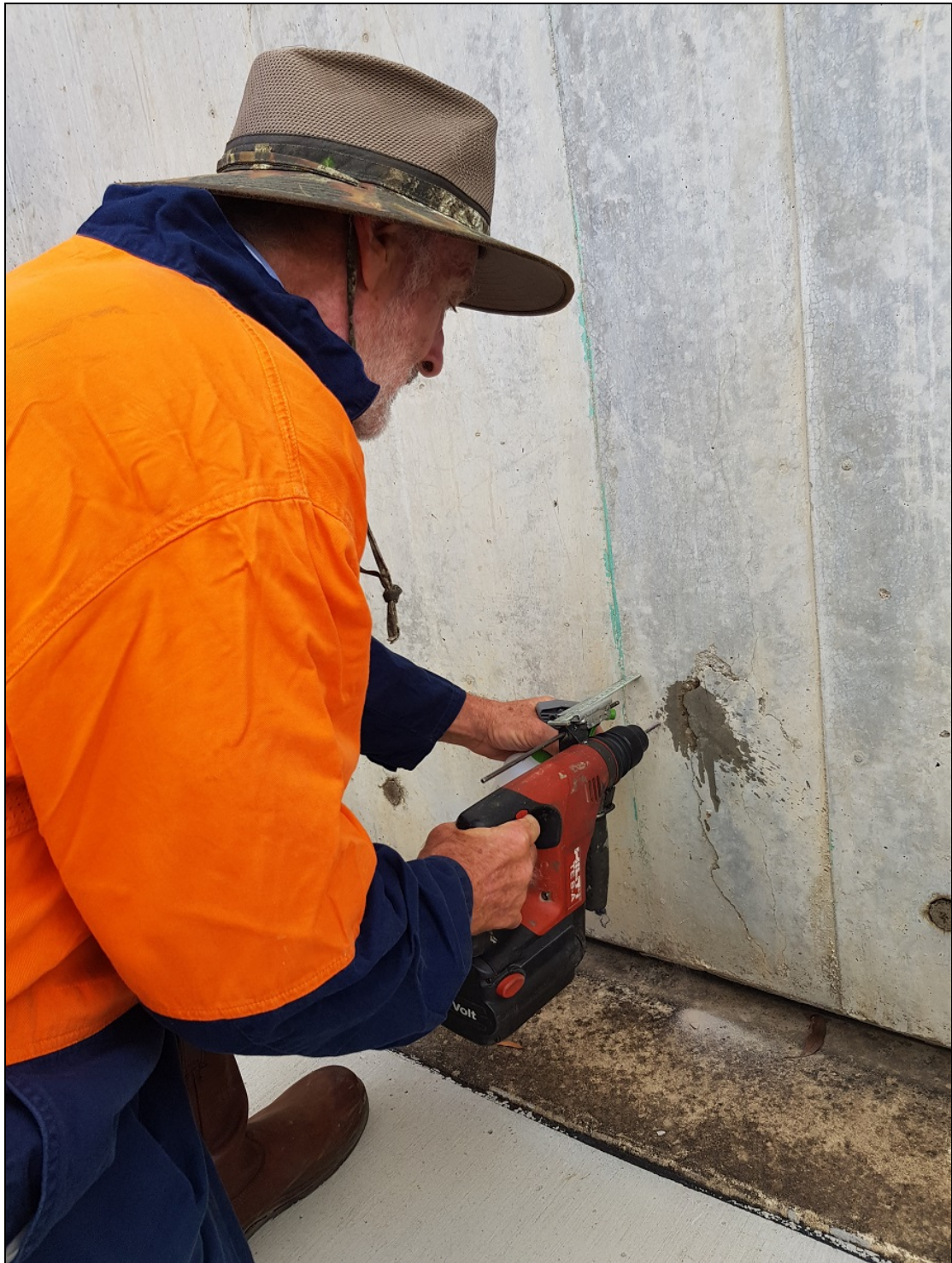
Figure 2: drilling holes in order to conduct carbonation deterioration depth
