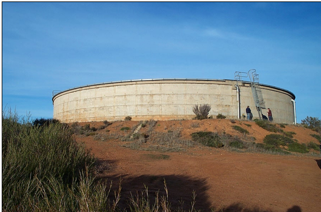
Figure 5 – SA Water’s Stokes WS119 tank
