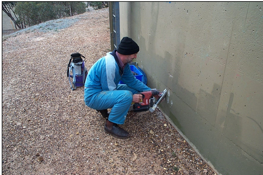
Figure 4: collecting a concrete dust sample for chlorides analysis
