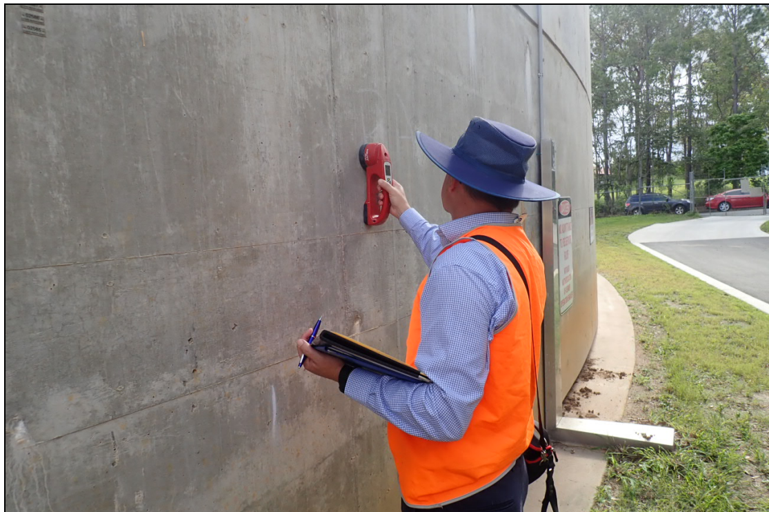
Figure 1: using a re-bar meter to conduct a steel cover depth assessment
