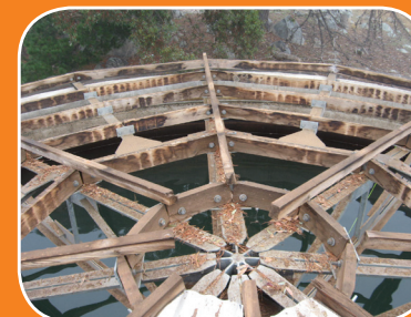
Centre pitched roof debris.
