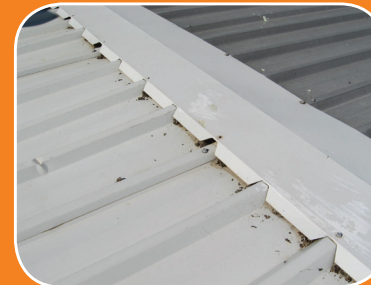
Ridge capping appears to be sealed.
