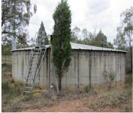
Trees starting to intrude onto storage tanks, causing roof impact damage or root intrusion
