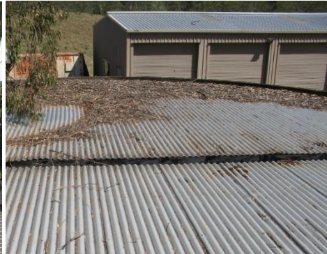
Overhanging trees allow vermin access to roof areas and deposit leaf debris
