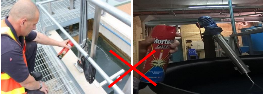
Spraying pests in close proximity to a water treatment process
