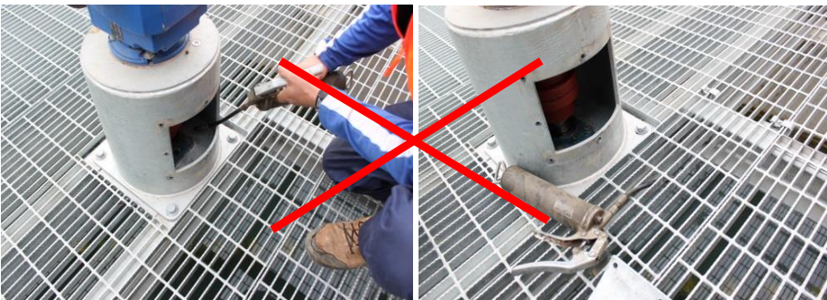
Grease gun being used directly over a treated water storage - note there is no provision to prevent any tools or materials entering the water
