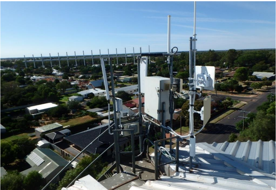
Aerials positioned over hatches and platforms on storage tanks encourage birds to roost and defecate over the surrounding area
