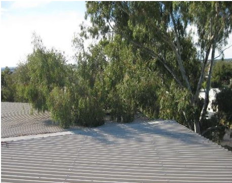
Overhanging trees allow vermin access to roof areas and deposit leaf debris
