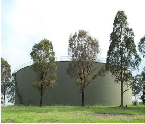
Trees starting to intrude onto storage tanks, causing roof impact damage or root intrusion
