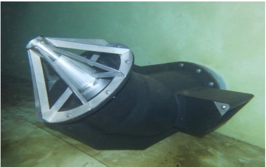
Two-way directional nozzles placed over common penetrations will mix the water without disturbing sediments
