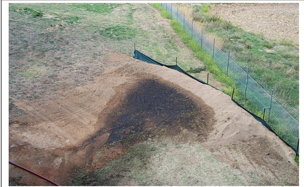
Figure 3 Course Sand Cofferdam after water has soaked away
