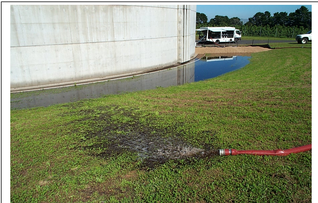
Figure 4 Tank Wall Cofferdam using coarse sand
