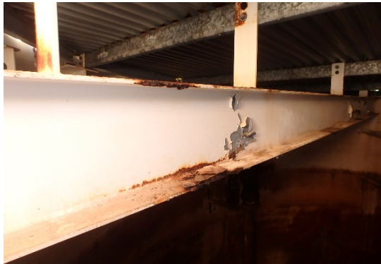
Severe corrosion on roof members or sub-standard light gauge components
