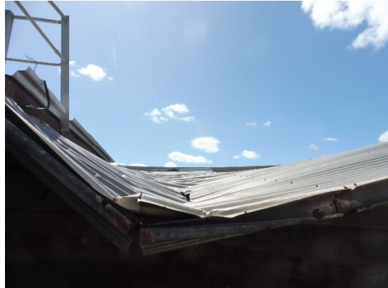
Severe corrosion on roof members or sub-standard light gauge components
