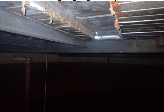
Severe corrosion on roof members or sub-standard light gauge components
